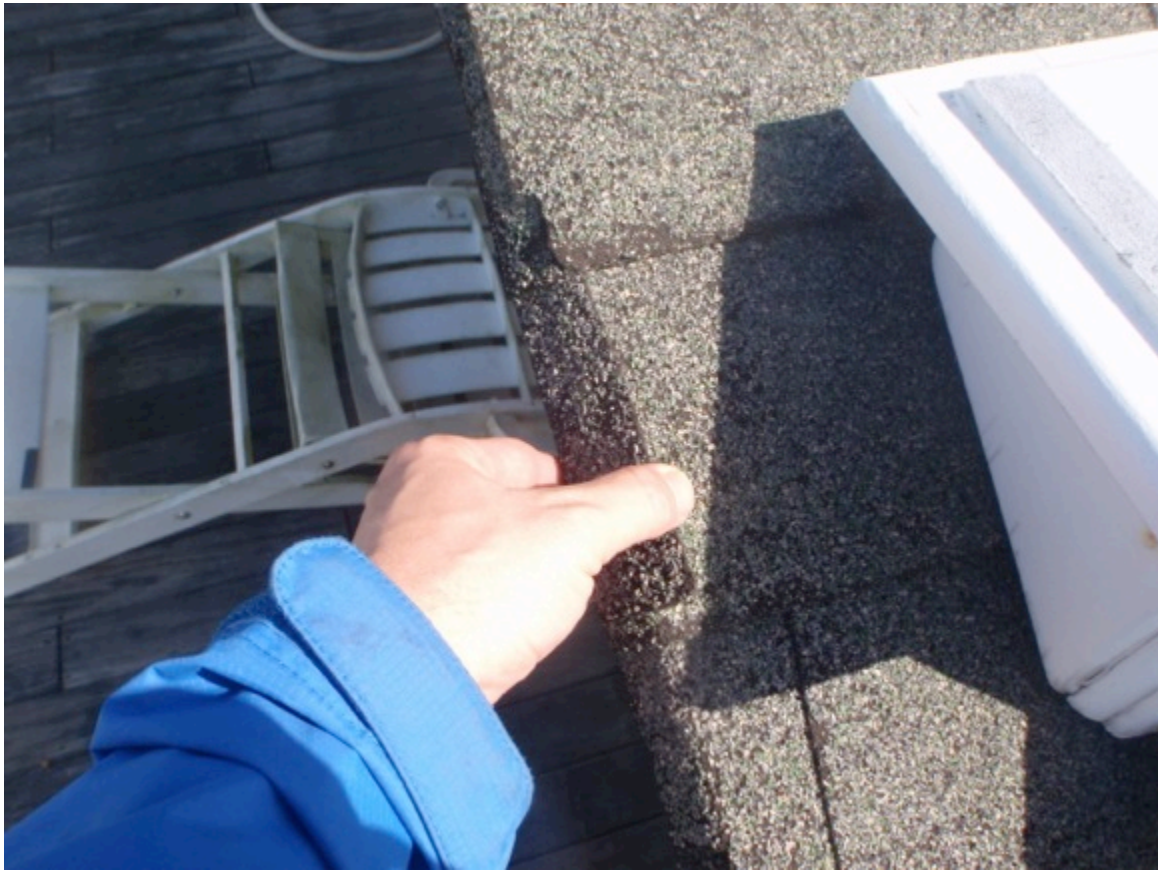
Multiple damaged shingle tabs were observed on roofline by fascia of top floor deck
