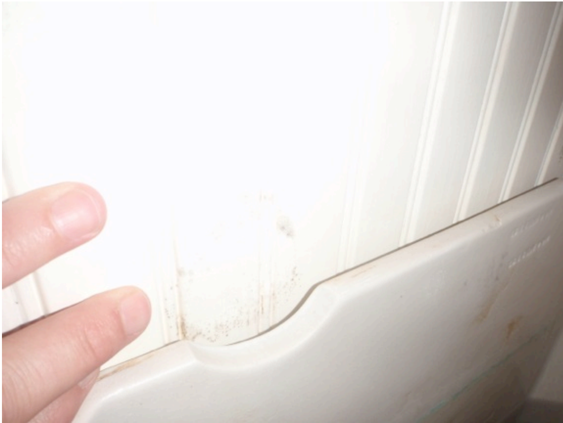
View of microbial growth presence observed on 2 nd floor hall bathroom behind toilet and ceiling sheetrock by fan above toilet
