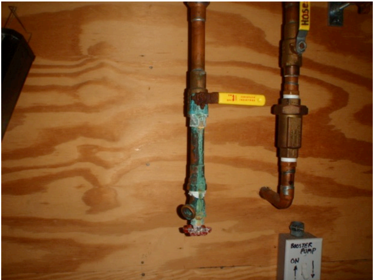
View of leaking handle and corroded handle observed at boiler room plumbing fixture at time of inspection
