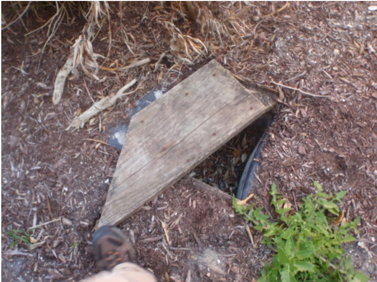
View of broken water meter box observed at right hand side yard water meter turn off meter/handle *Trip Hazard
