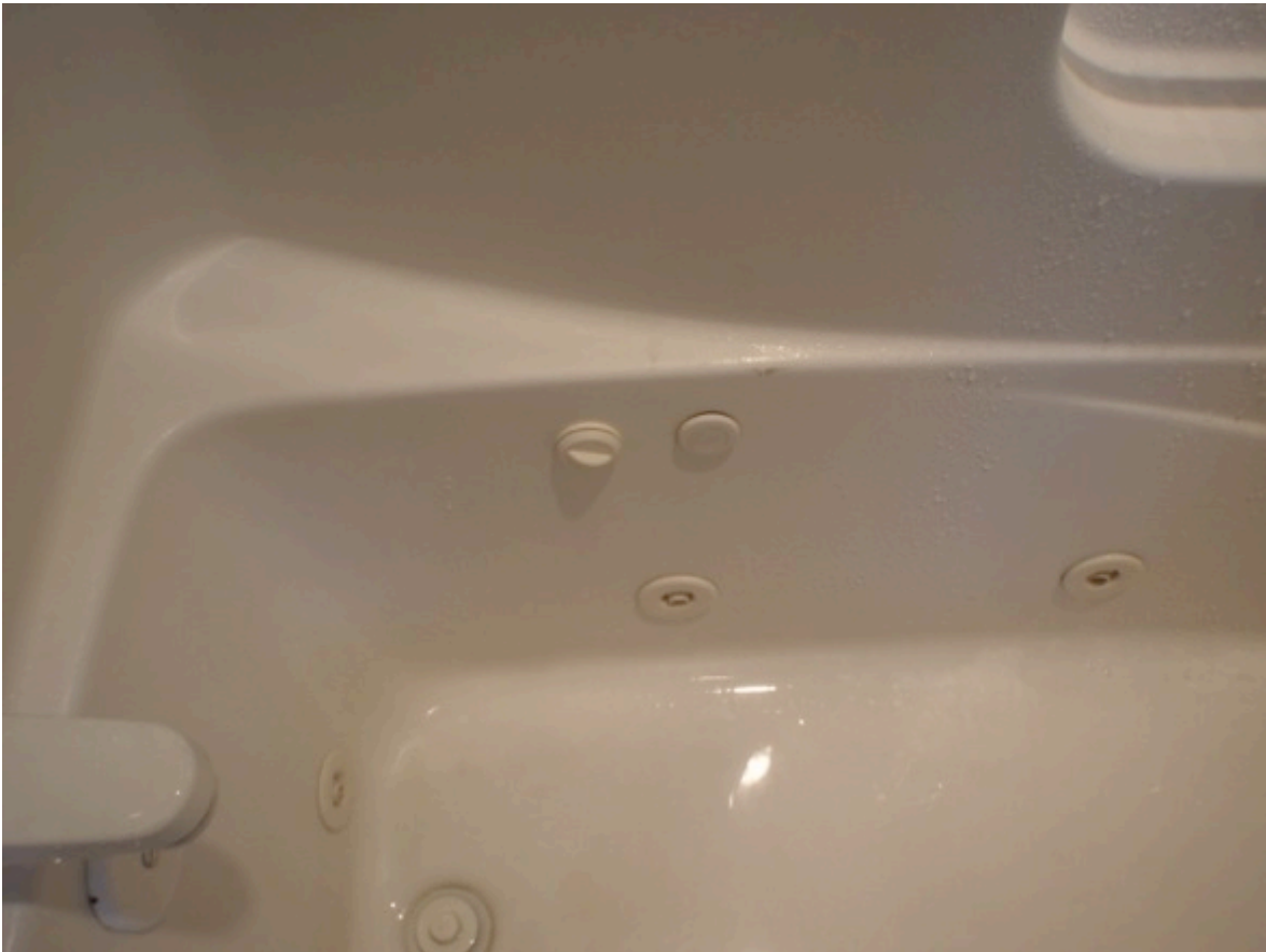
2 nd floor Whirlpool jets kept tripping breaker in carport breaker panel box at time of inspection
