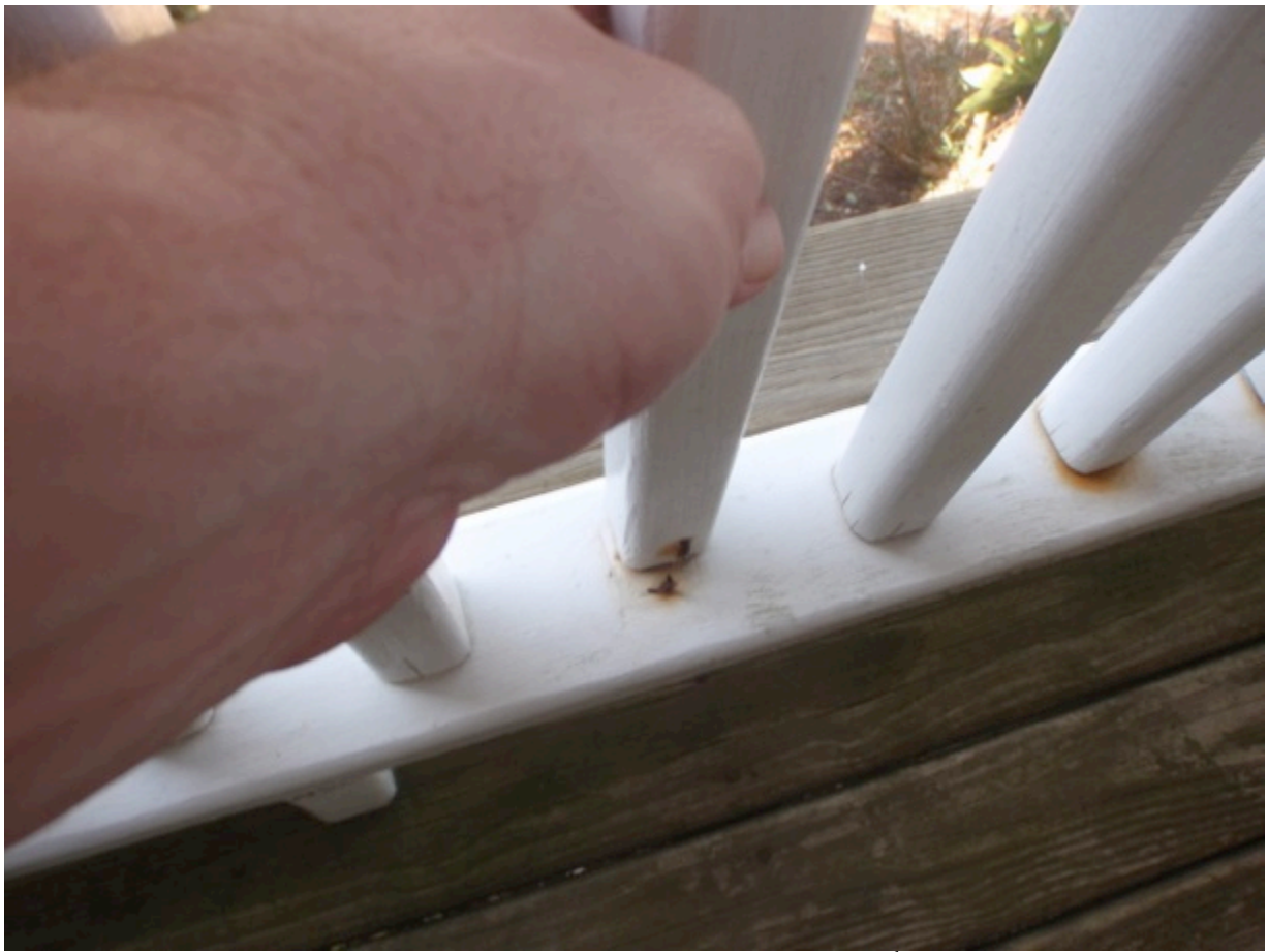
View of rusted out fastener nails and loose railing pickets observed on 2 nd floor main house deck railing
