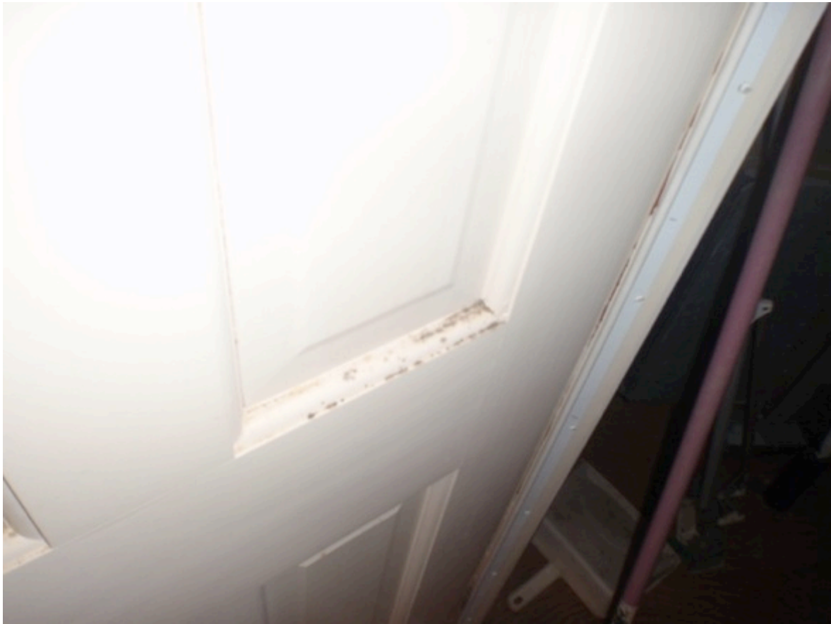
View of mildew/microbial growth exposure was observed on the back of top floor attic access doors
