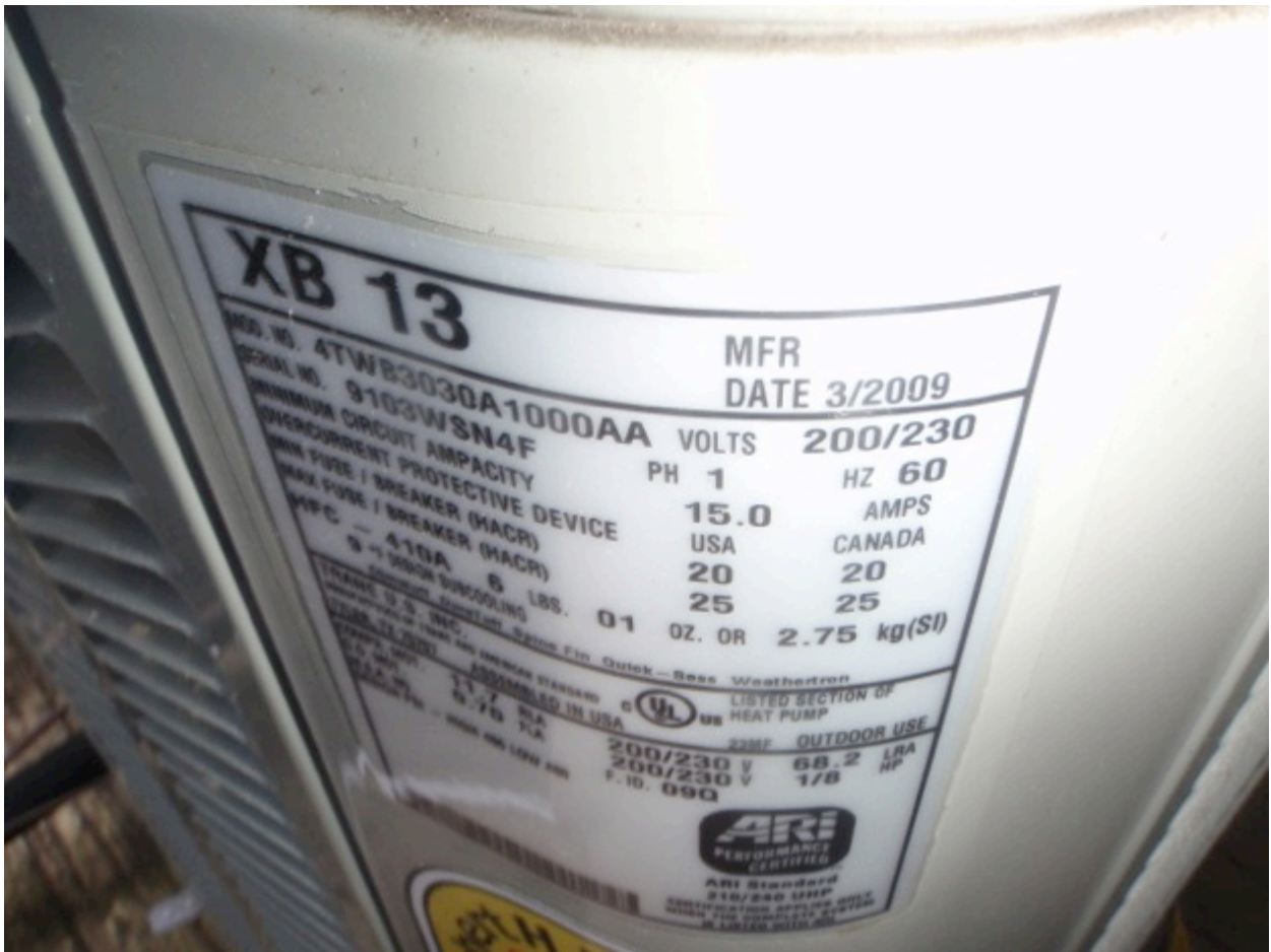
4 out of five HVAC heat pumps were updated in the 2000's, one is original
