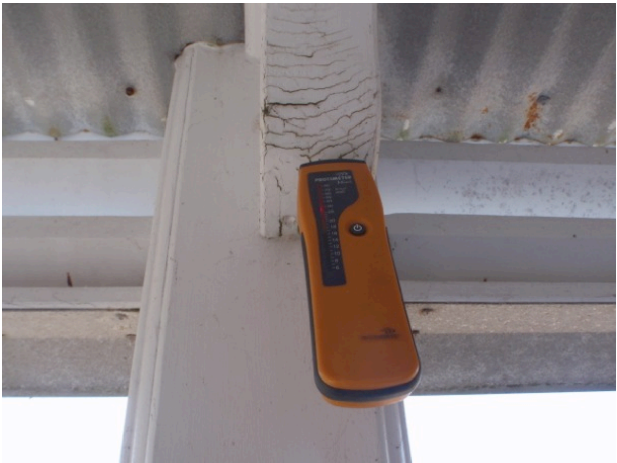
View of moisture exposure/damage at sound side porch 3 rd floor framing detail
