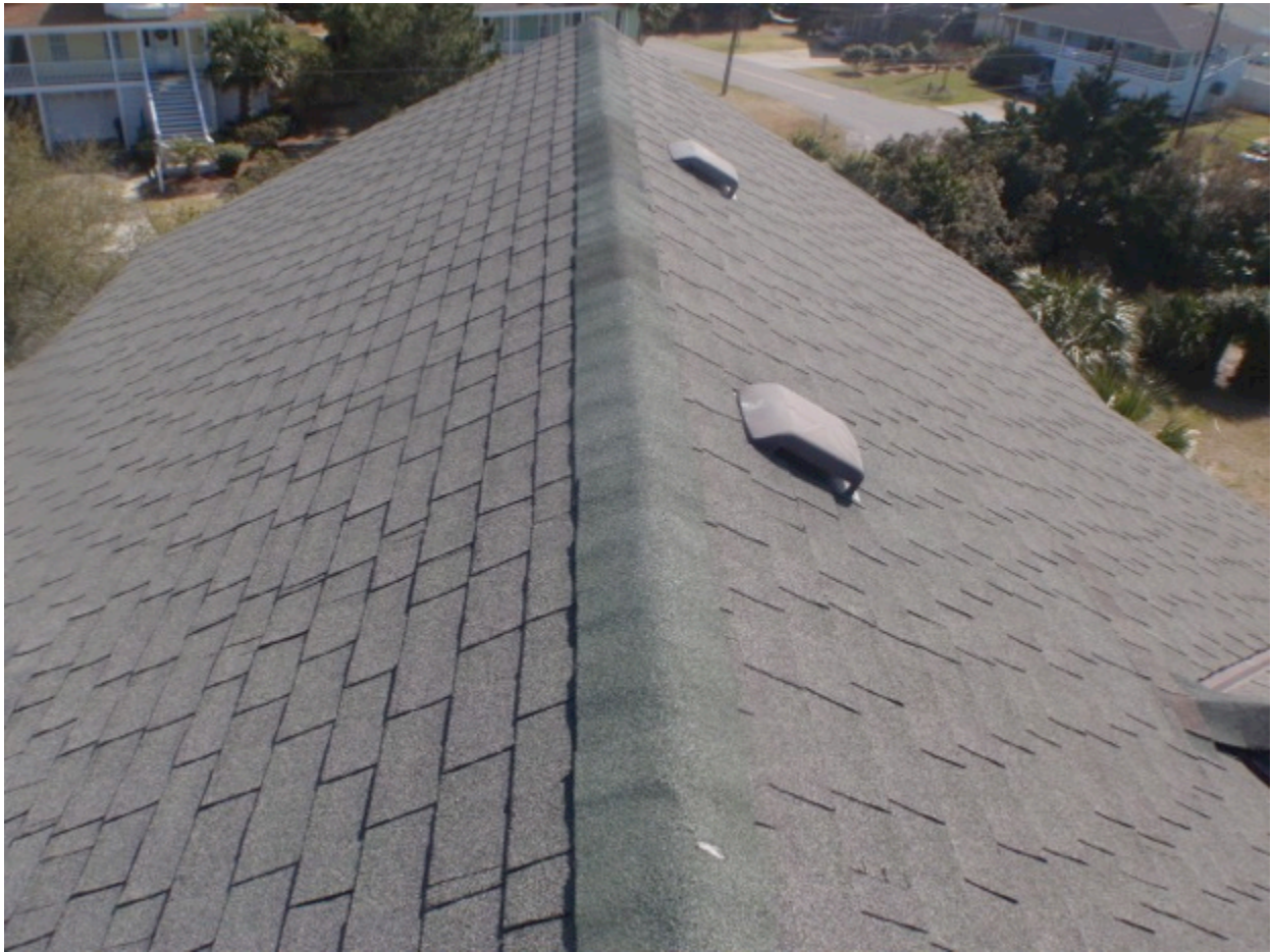
Walk on roof view-Original shingle tabs
