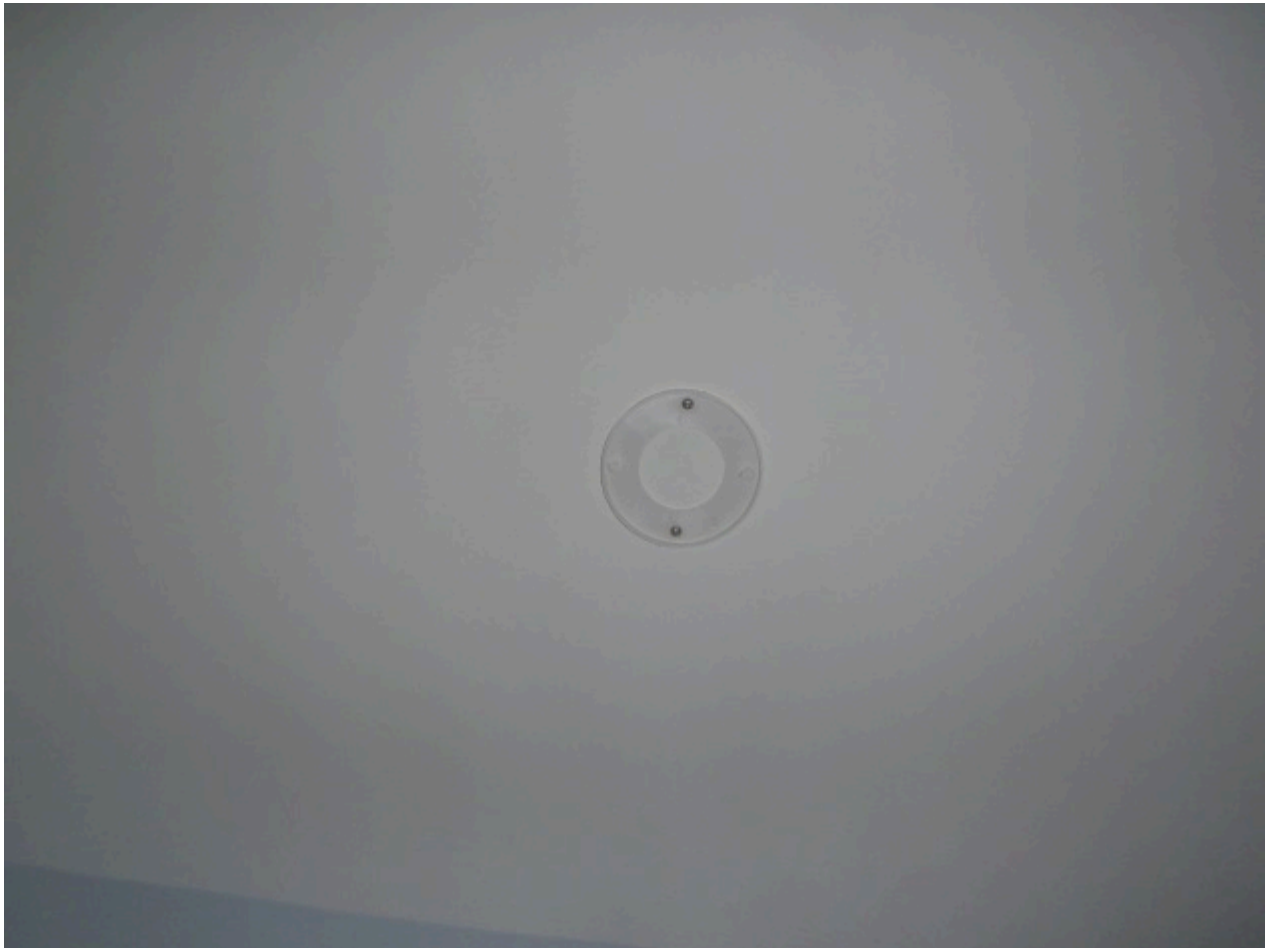
View of missing smoke detector observed on 2 nd level of home, see summary page comments concerning homes smoke detectors
