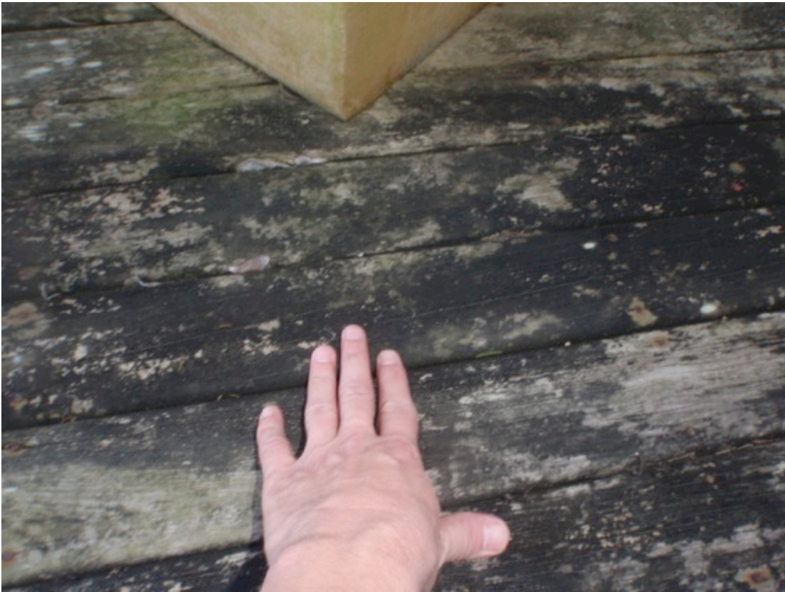
Top floor sound side deck boards are in poor condition and need repairs soon by a qualified contractor
