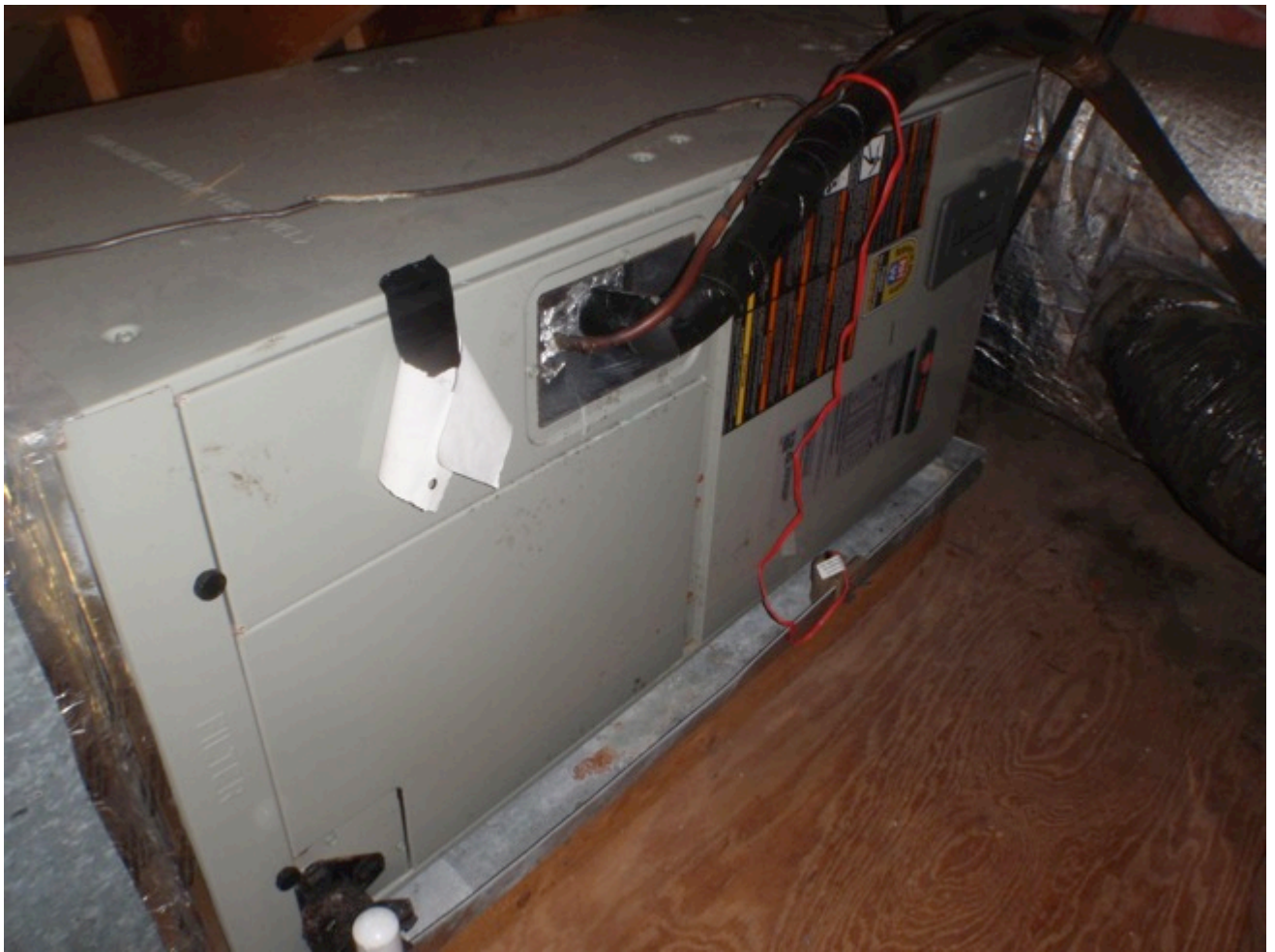
View of attic HVAC air handler in above view
