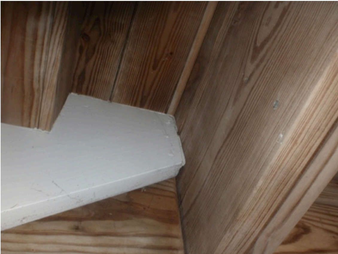
Exterior stair stringer support boards that tie into band joist at deck platform framing need ledger strip or joist hanger supports added to properly support stairs runs on home *Old code compliant
