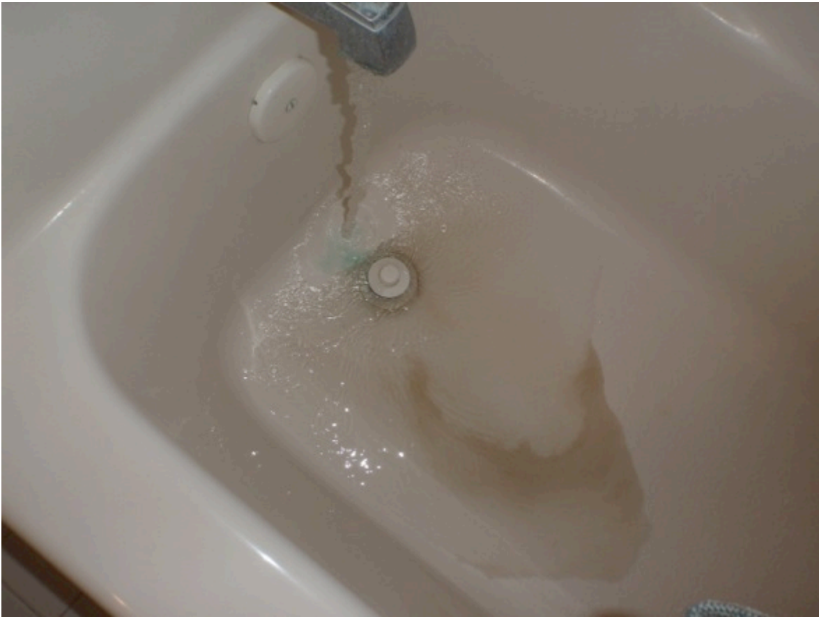
View of dirty fixture water was emitting from homes plumbing (copper vs. lack of use)
