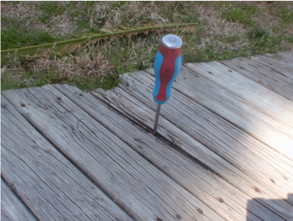
Plank walk boards at back patio are in need of repair *multiple
