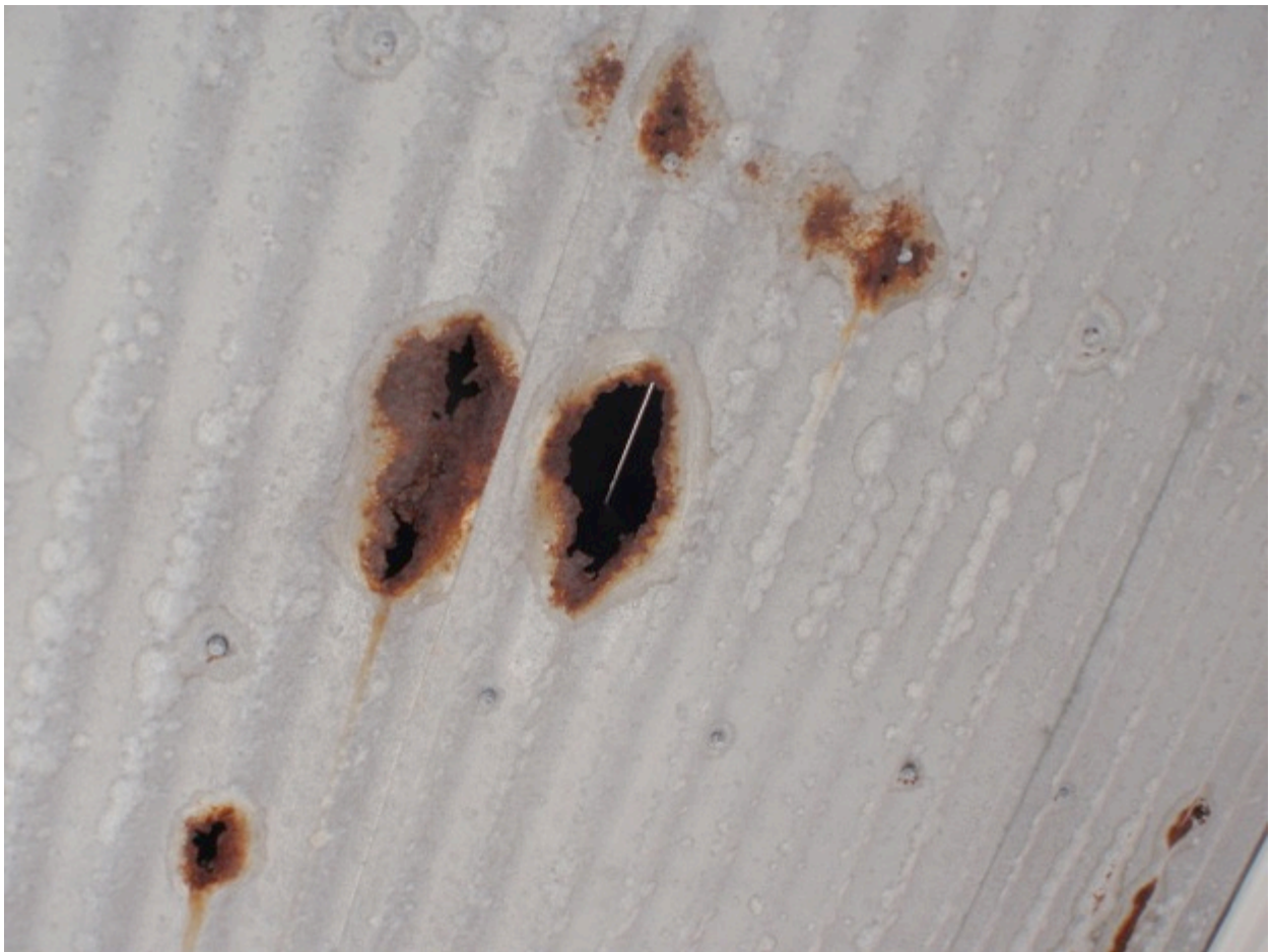
All deck overhang rain water diverters need to be replaced on all deck underpinning on sound side of home
