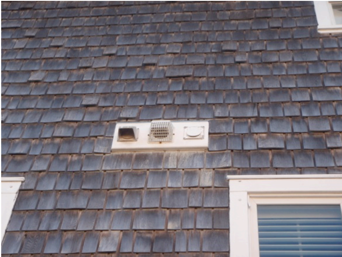
View of missing side yard bathroom vent fan cap, also note window shifted shingles and weathering of original tabs
