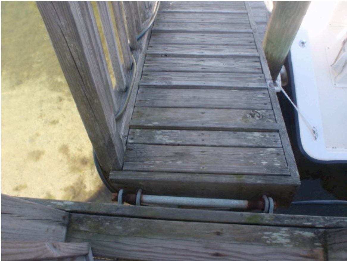
Gazebo to floating dock transition needs securing repairs by contractor
