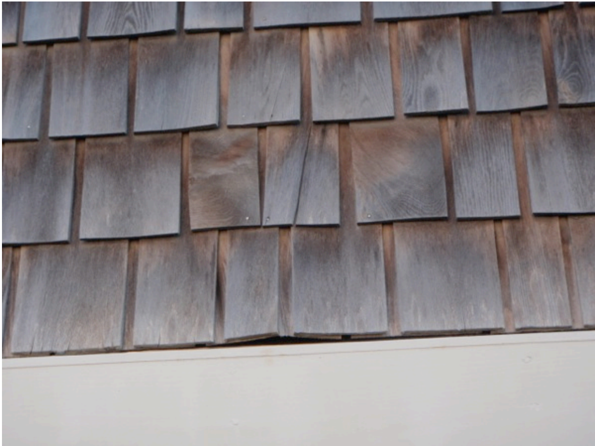
View of original cedar siding observed on exterior cladding of subject home, note numerous past nail securing repairs have had to be added to secure loose shingles over the years
