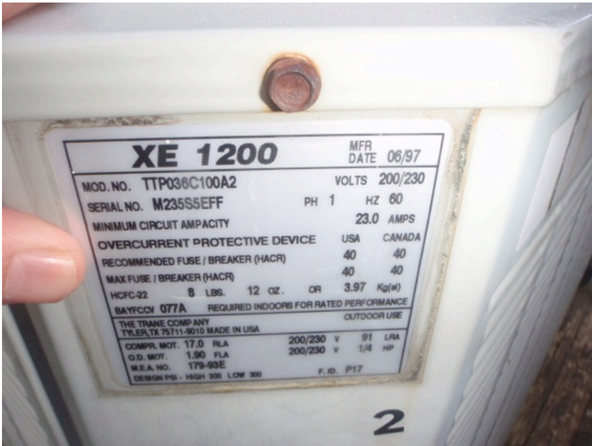
View of original HVAC unit observed for subject home, only one out of four systems has not been updated
