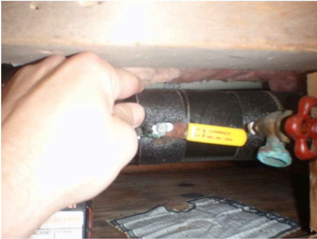
View of leaking/corroded water line turn off handle observed at carport side shed
